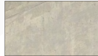
Exposed: Sealed Epoxy Concrete
